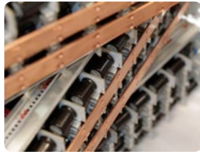
Fig. 5. Copper busbars.
